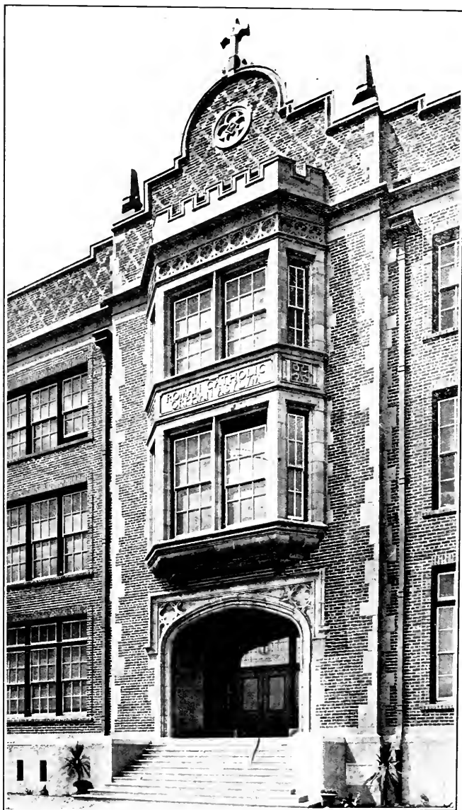
CENTER BAY, ROMAN CATHOLIC ORPHAN ASYLUM, SAN FRANCISCO SMITH O'BRIEN, ARCHITECT A LATE EXAMPLE OF GOOD BRICK WORK
